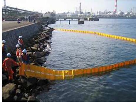
Oil fence installation drills at Toray's Chiba Plant
