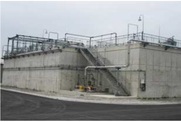
New MBR treatment facility at the Toray Tokai Plant
