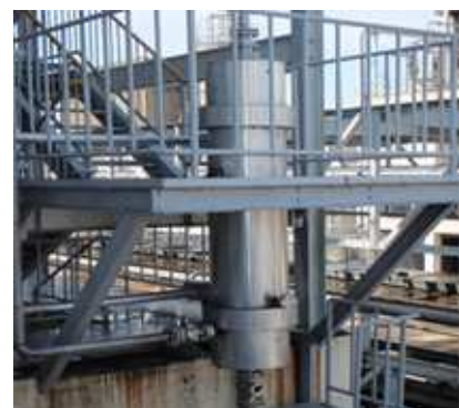
Device for the collection of organic exhaust gases installed at Toray Plastics (Malaysia) Sdn. Berhad
