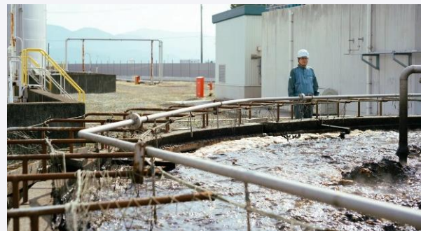
Wastewater treatment using the activated sludge method
